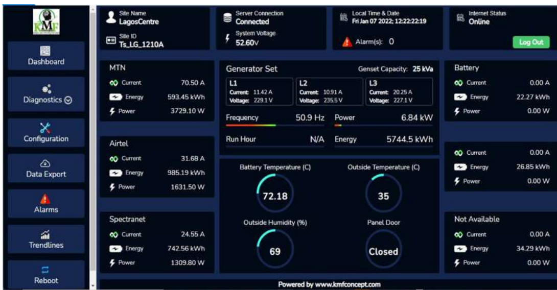
Figure 29. Remote monitoring agent (RMA) local dashboard.
